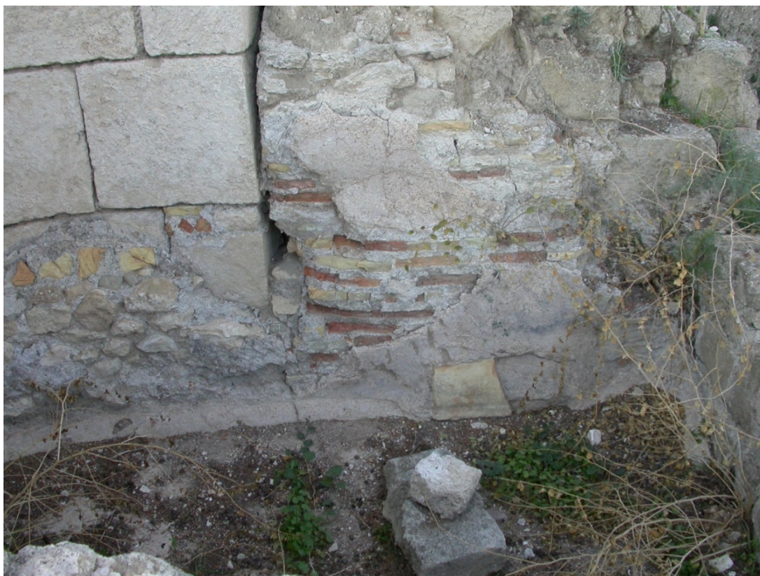
Fig. 7. Temple of Zeus, Salamis-Constantia (Cyprus). Fountain in the eastern wall, looking north. Note the difference between the Roman ashlar masonry on the left with the Byzantine brickwork on the right (author).
