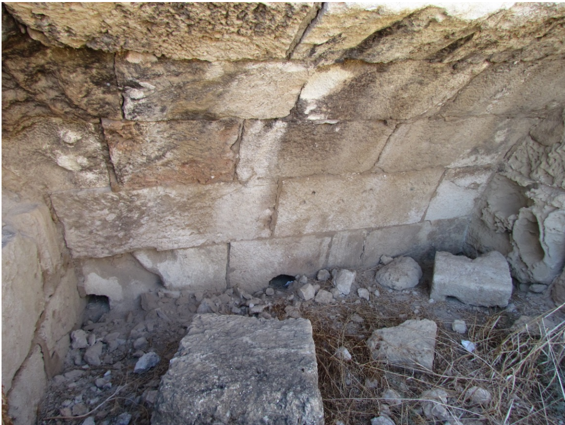
Fig. 10. Loutron, Salamis-Constantia (Cyprus). Byzantine renovation phase: settlement chamber between reservoir and barrel-vaulted passage (author).
