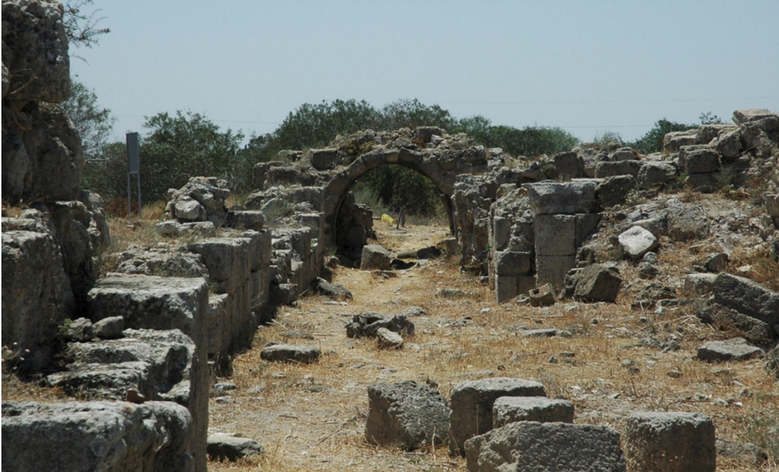
Fig. 9. Loutron, Salamis-Constantia (Cyprus). Byzantine renovation phase: barrel-vaulted passage between earlier façade (right) and later wall (left) (author).
